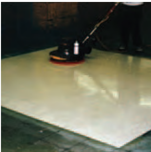
3 - the high gloss of the restored floor finish is similar to that of the tile when it is newly installed
